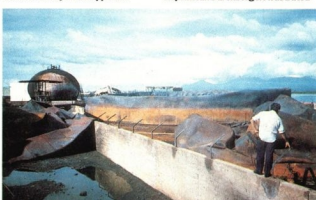
Ravaged oil depot at Corinto: a CIA raid by "unilaterally controlled" latinos
